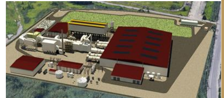
1,300 t/d rotary kiln gasifier with HTL
