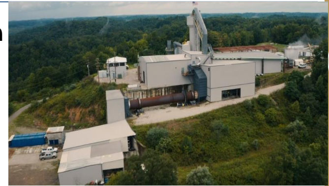
440 t/d rotary kiln MSW gasifier
